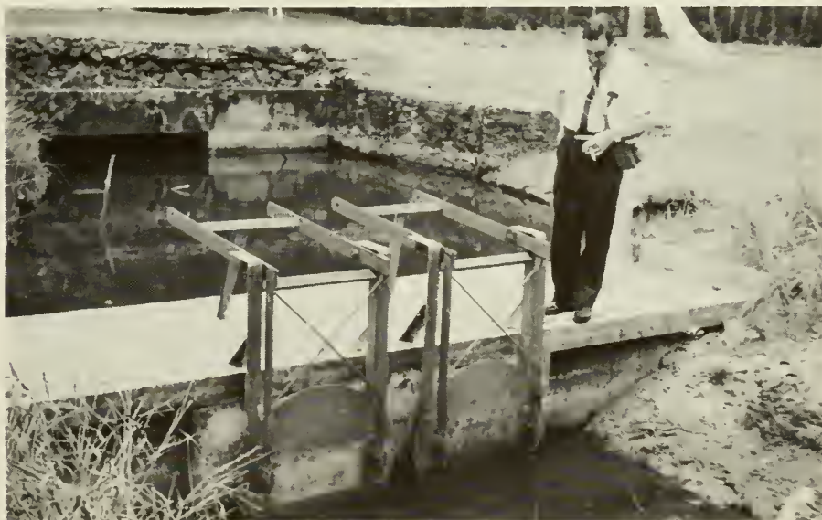
John Palmer Smith, former Chief of the Division of Sanitation, who initiated sandfly control research here, inspects a tide gate installation at Coco Solo.
